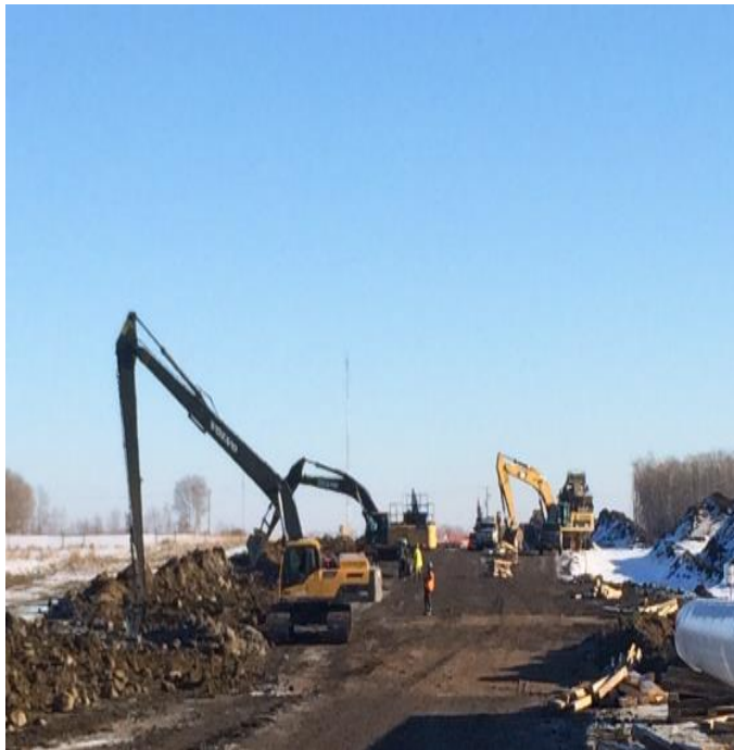
777 + 900 Jackson Creek area Mainline backfill and pipe shading.
