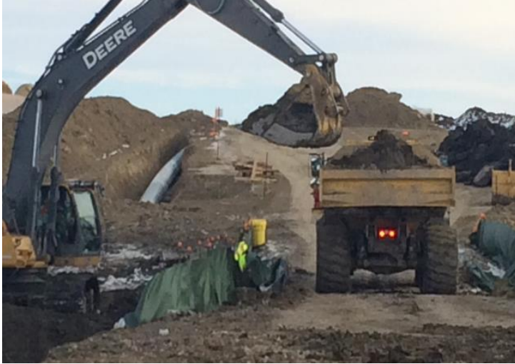
Montgomery Creek SK WC 79 excavating ditch and tying in pipe.
