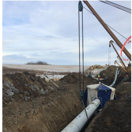
Montgomery Creek SK WC 79 excavating ditch and tying in pipe.
