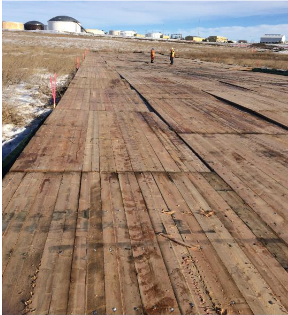
Pipe Stone Creek - Geo tech fabric and matting laid over area for equipment workspace & Track bore bay backfilled.
