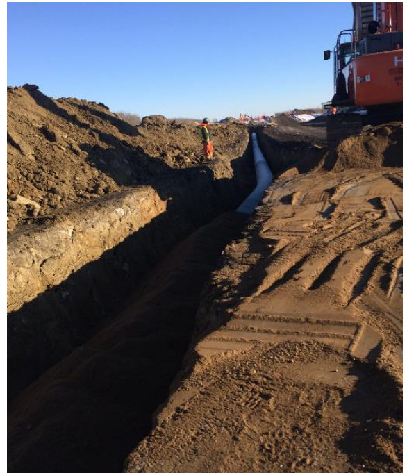
777 + 900 Jackson Creek area Mainline backfill and pipe shading.
