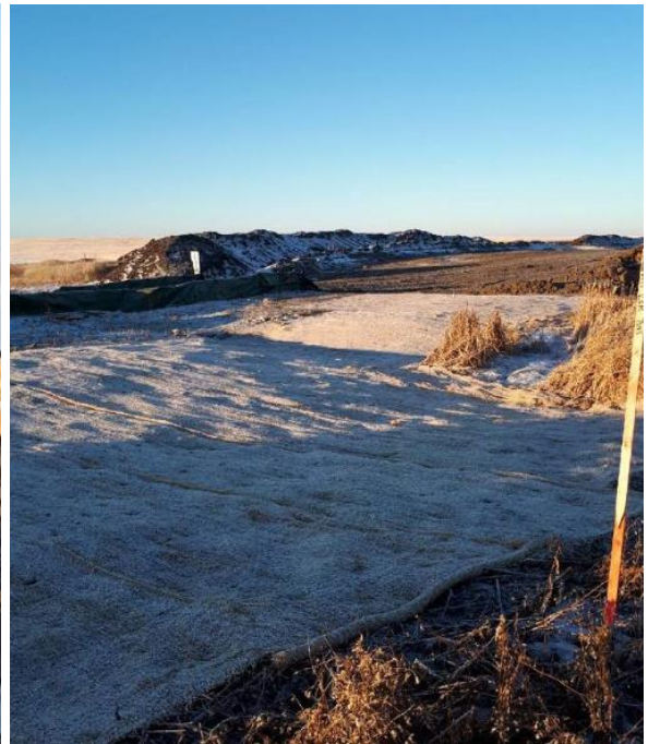
Montgomery Creek SK WC 79 backfilling ditch line and erosion blanket placed over seed mix.
