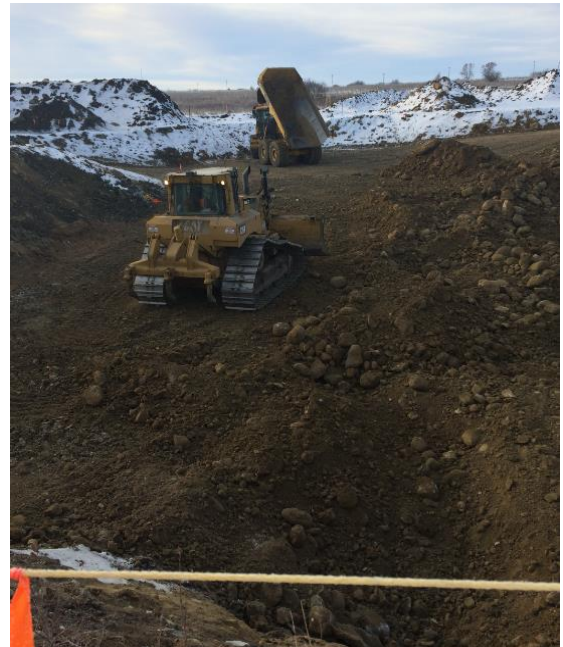
Pipe Stone Creek - Geo tech fabric and matting laid over area for equipment workspace & Track bore bay backfilled.
