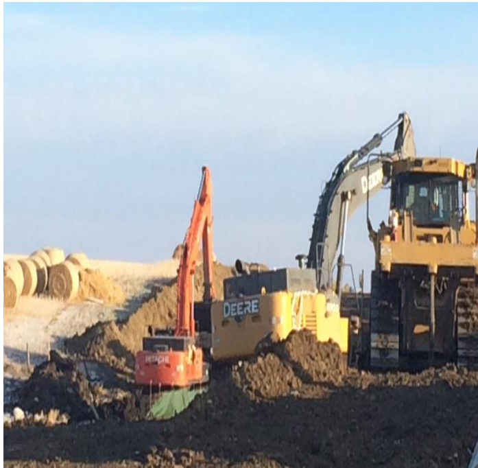
Montgomery Creek SK WC 79 backfilling ditch line and erosion blanket placed over seed mix.
